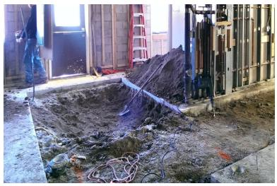
Are we still making progress? Rebuilding is pretty serious when the bathrooms go away. Last week we ripped one out to make way for the concrete cutters. They sliced up a big section of floor to lay in some new drain pipes.
